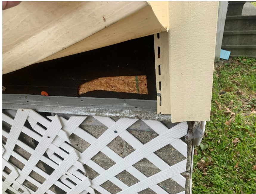
Photograph No. 9 HA-09: Black Tar Paper Vapor Barrier
