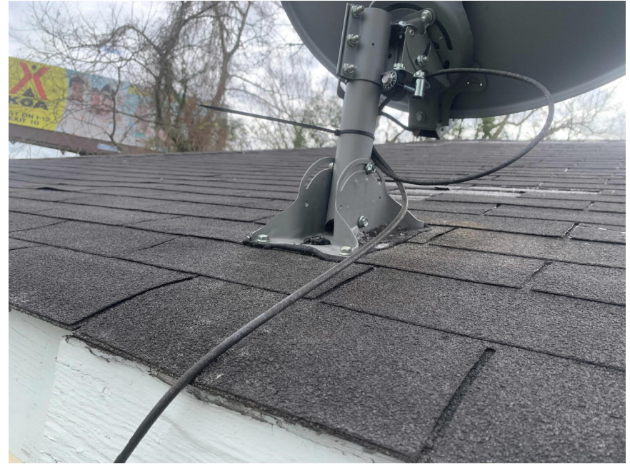
Photograph No. 8 HA-08: Black Roof Shingles with Black Tar Paper
